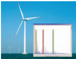
Remote monitoring and diagnosis
